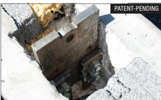
Patterson's Sandwich Anchor installed
