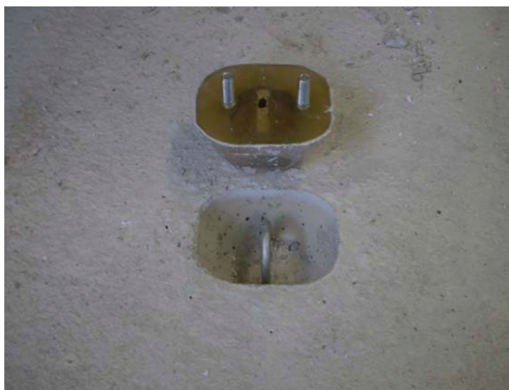
Figure 1 - A.L. Patterson precast anchor (with recessing device removed)
