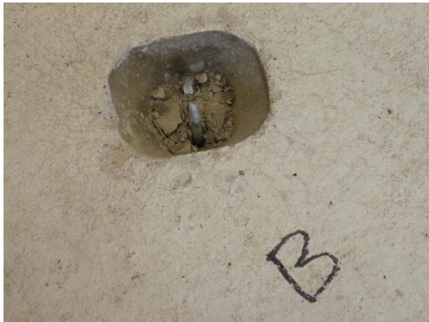
Figure 5 – Sample B Failure
